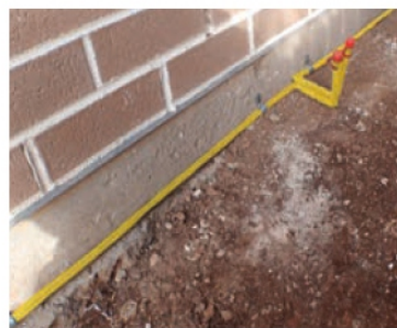
Pipe clipped low on footing
