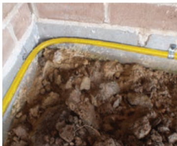
Pipe clipped high on footing
